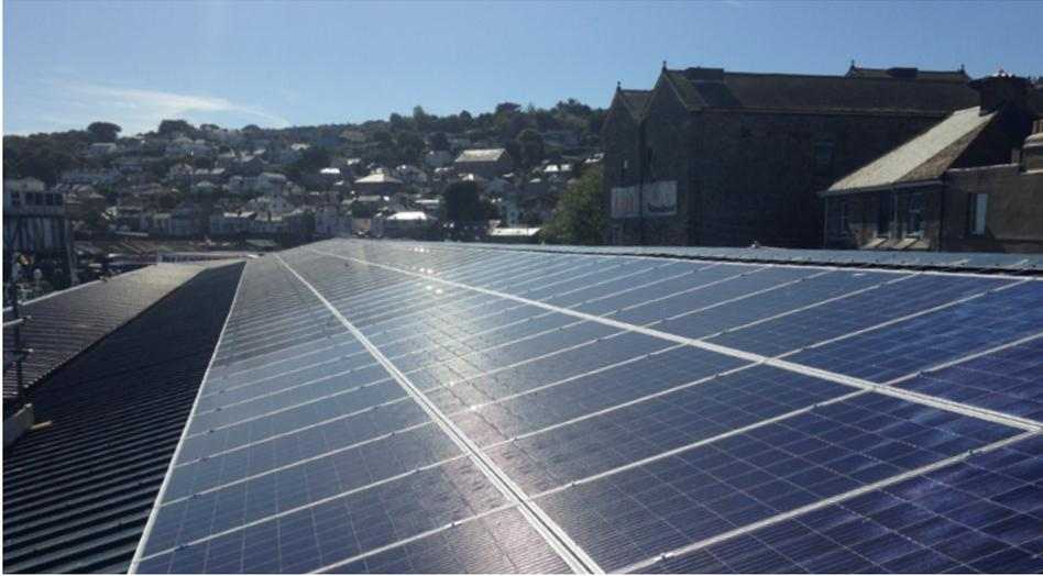
Following CNE's and CPC's support, a 150kW PV array was installed on the roof of Newlyn Fish Market. The system has the ability to monitor each individual panel and sits on its own string; this was deemed essential to limit system losses through interaction with the local seagull population. It is expected that 78% of the energy generated will be used on-site, saving 38.6 tonnes of CO<sub>2</sub>e per year.
